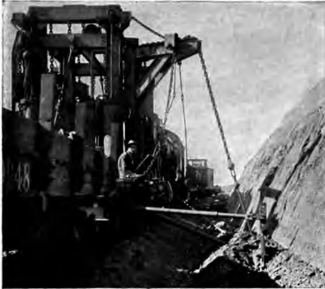
Bowman Ditcher Plowing Ditch
